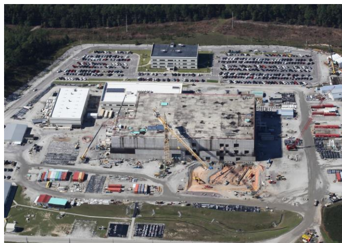
photo: Mixed Oxide Fuel Fabrication Facility (MOX plant) under construction at SRS; rumors of construction problems are constant, DOE testified to Congress on October 7, 2015 that the "reinstallation" rate for items improperly installed was 25%; ©High Flyer, special to SRS Watch, taken October 1, 2015
